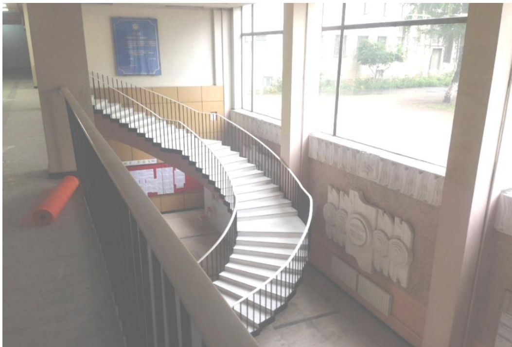
Fig. 3.42. Monolithic reinforced concrete stairs designed to connect the lobby with the second floor between axes "B-H", "2-4" at elevation +3.900
