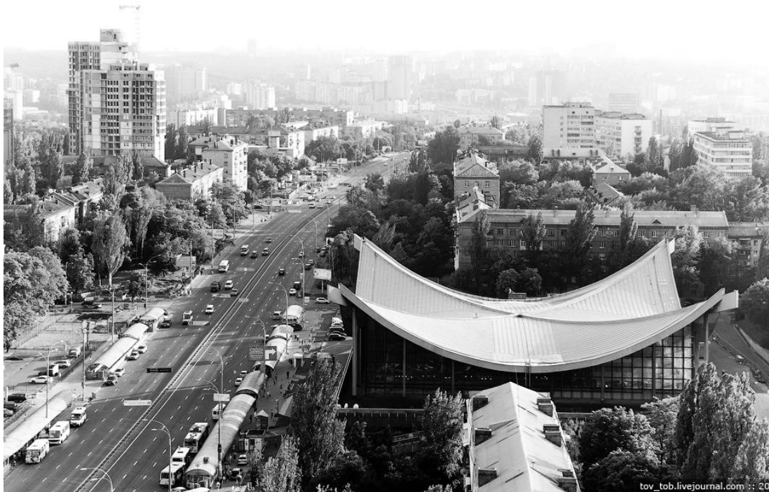
Fig. 12.11. Example of a building with a suspended roof using rigid cables: Furniture Exhibition Store, Kyiv, 1975, Architects: N.B. Chmutina, Yu.A. Chekanyuk, Building dimensions: 63.0 × 63.0 m
