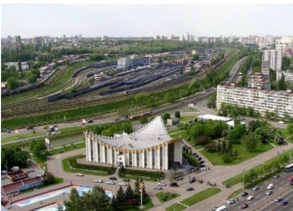
Fig. 12.9. Example of a building with a suspended shell roof of negative gaussian curvature:
