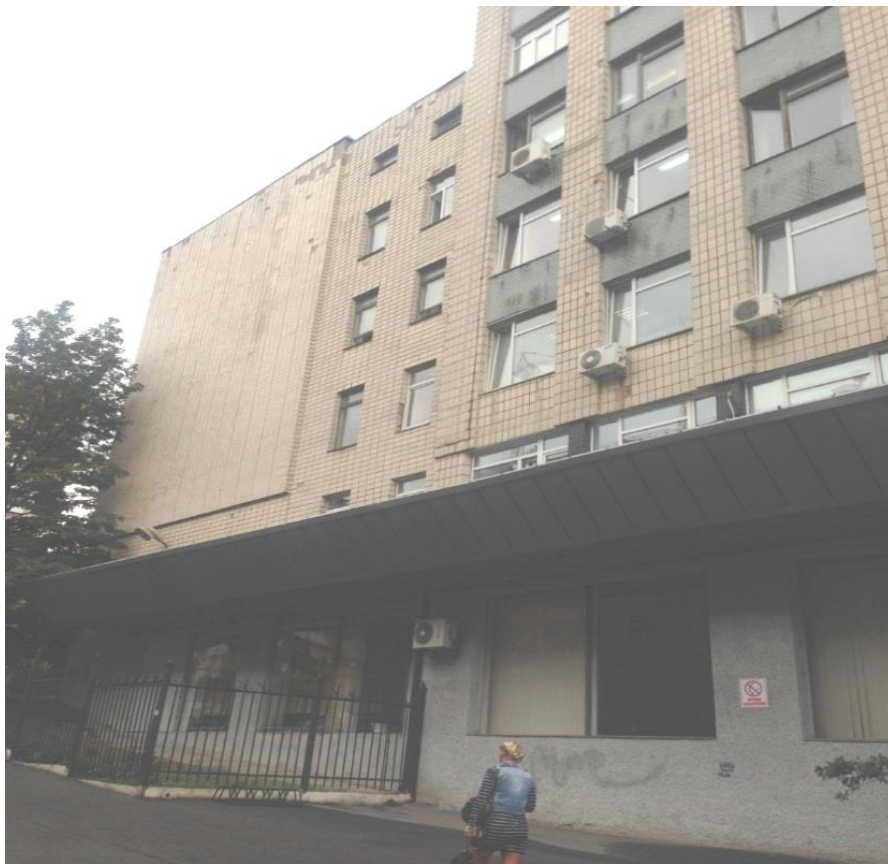
Fig. 3.39. Fragment of the facade of building "B" in axes "1–3"
