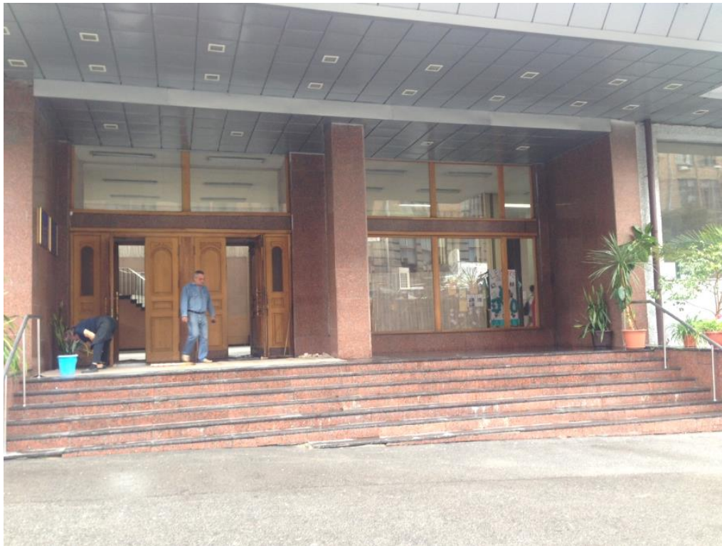
Fig. 3.38. Entrance area of building "B" in axes "3–5"
