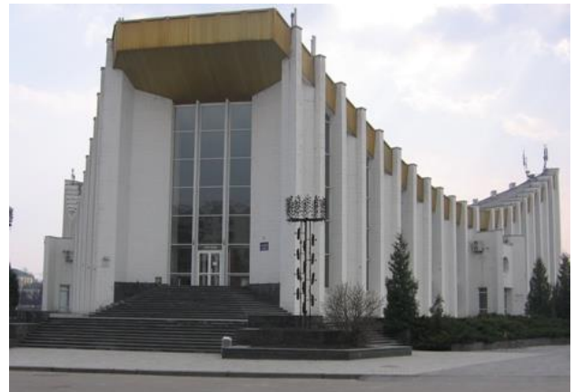
Fig. 12.9. Example of a building with a suspended shell roof of negative gaussian curvature:
