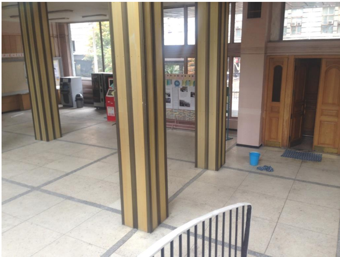
Fig. 3.40. Lobby area of the building in axes "3-5", "A-B" at elevation -1.100
