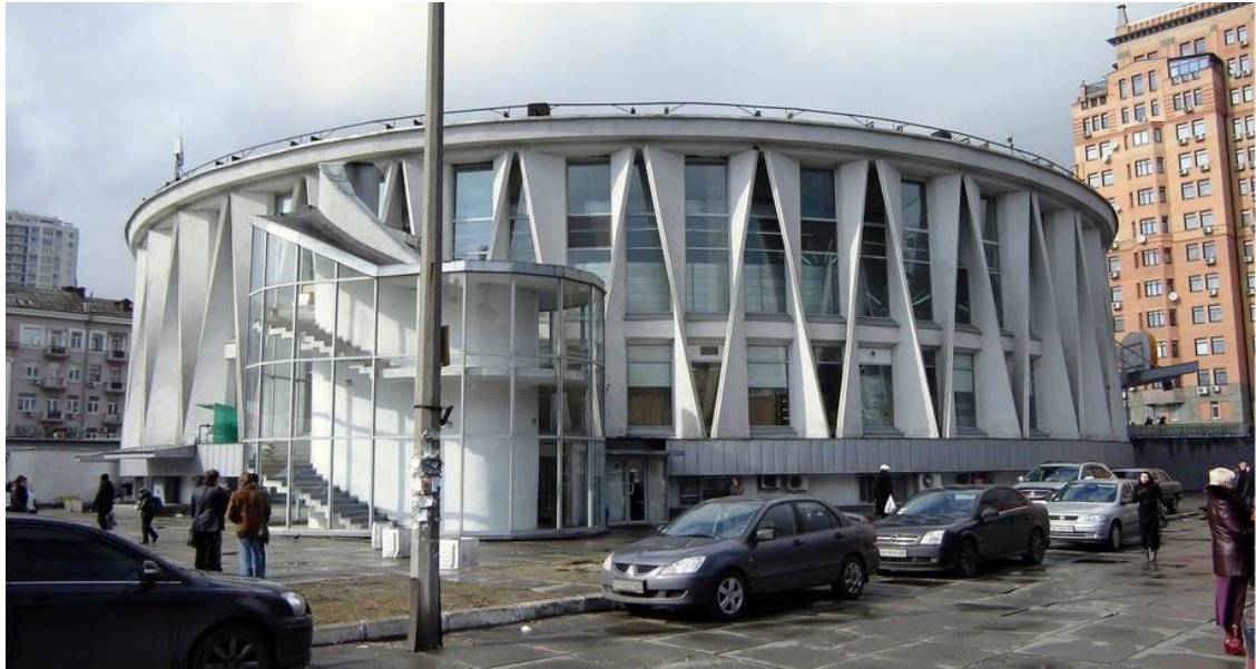
Fig. 12.10. Example of a building with a suspended roof system for a hall with a diameter of 51.8 m and radially arranged cables: shopping mall in Pechersk, Kyiv, 1982, Architect: A.M. Anishchenko
