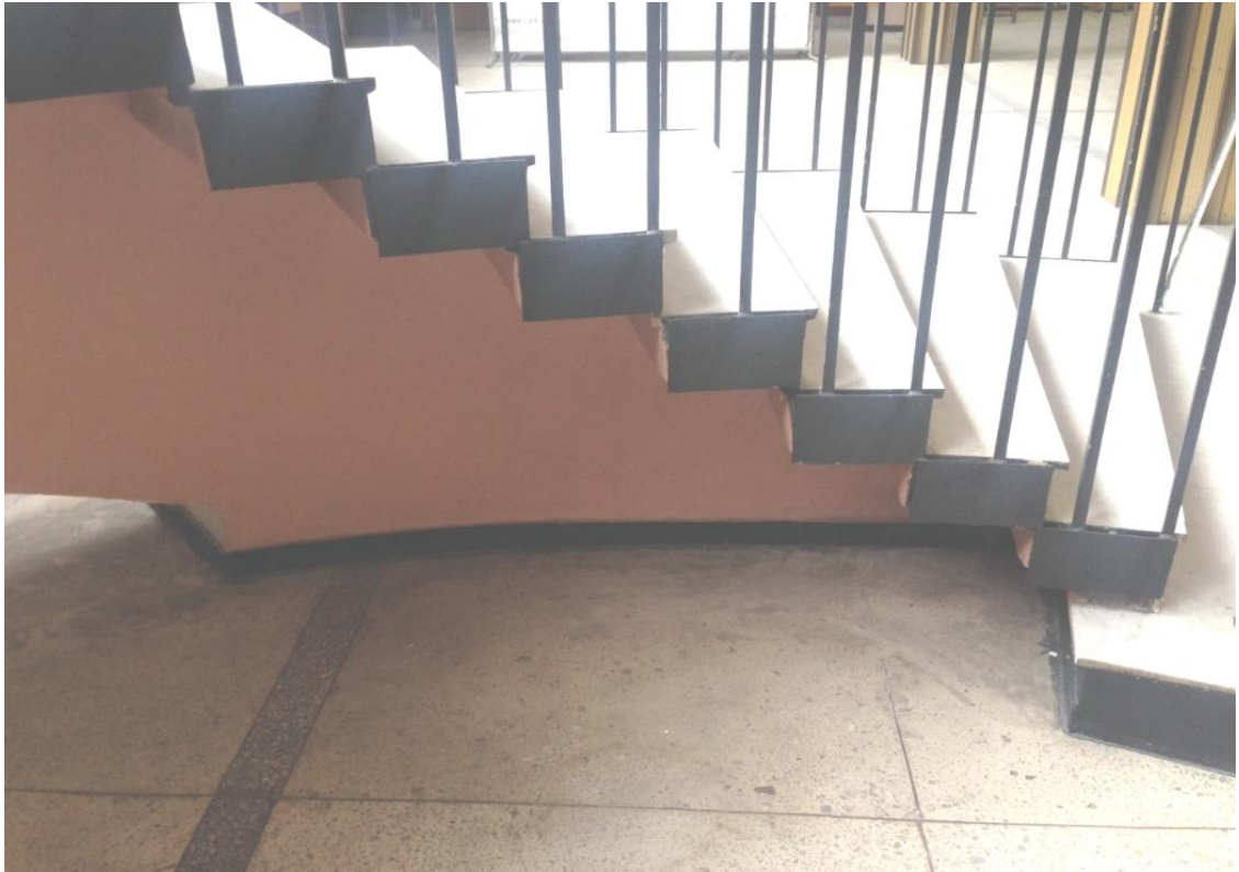
Fig. 3.43. Support of the curvilinear supporting beam on the monolithic reinforced concrete slab between axes "3-4", "B-H", at elevation -1.100
