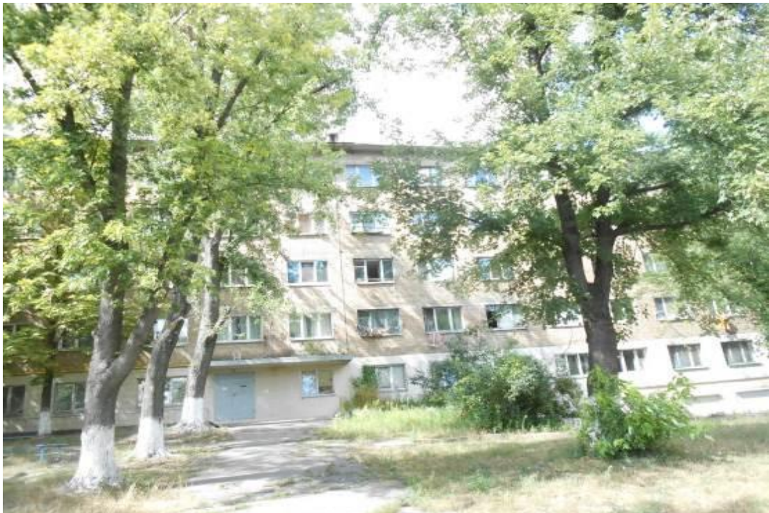
Fig. 3.19. Fragment of the main facade along axis "A" between axes "1-6"
