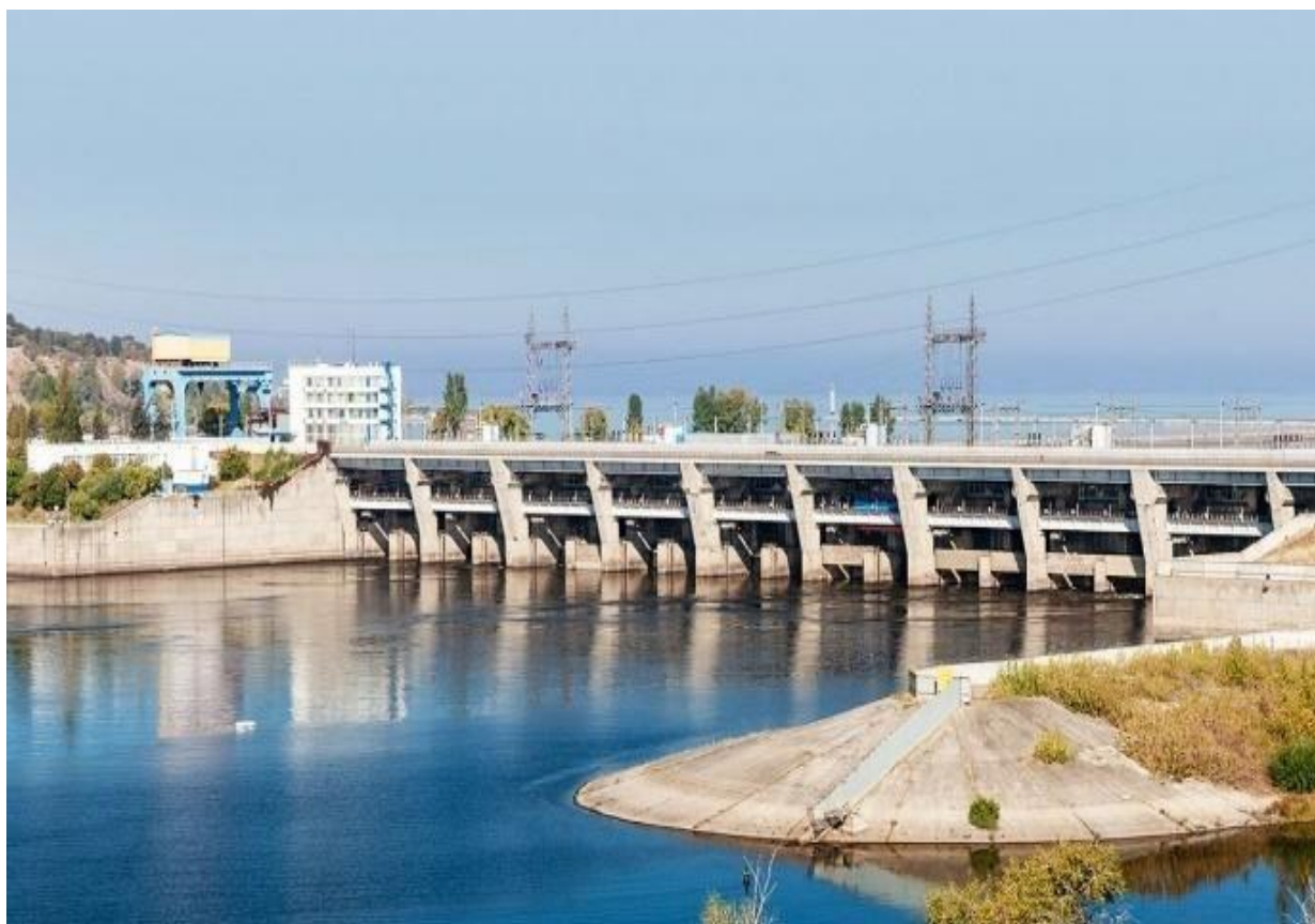
Fig. 2.7. Kyiv Reservoir embankment*
