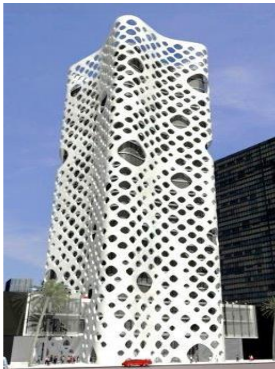
Fig. 1. Building in the form of an "Exoskeleton", Dubai
