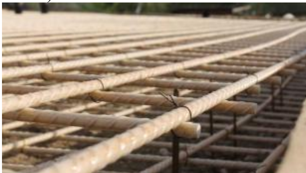
Fig. 3. Example of composite reinforcement application
