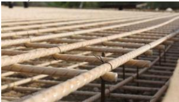
Fig. 3. Example of composite reinforcement application
