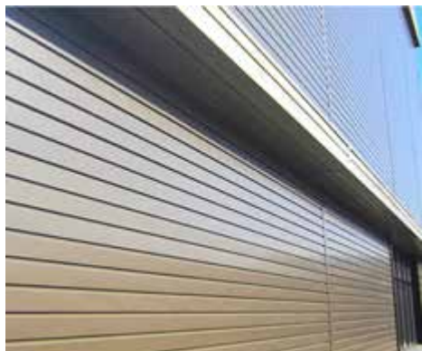
Fig. 4. Facade decoration with siding
