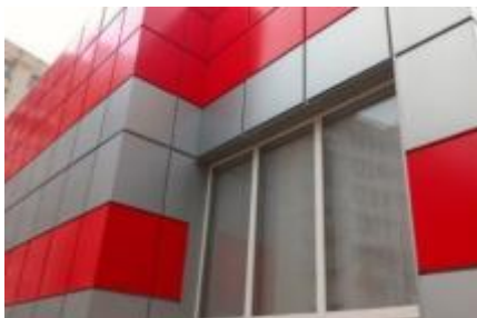
Fig. 6. Facing the building with facade cassettes
