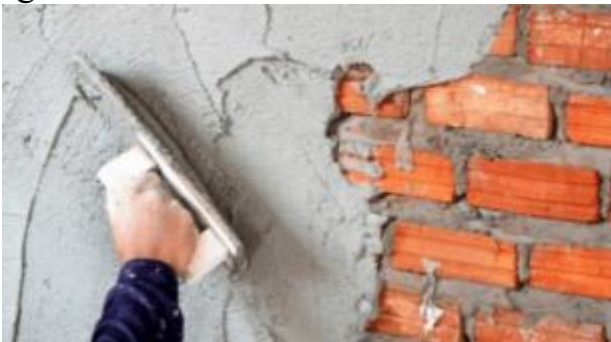
Fig. 2. Plastering the facade
