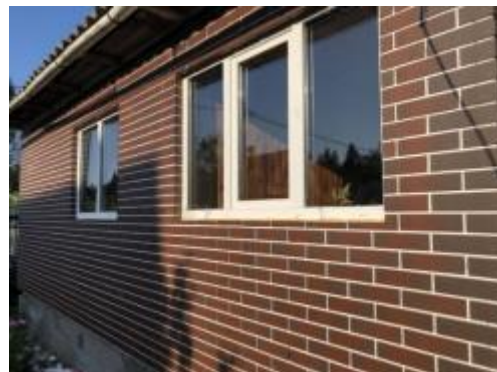
Fig. 5. Facing the facade with ceramic tiles
