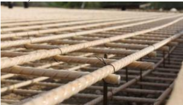
Fig. 3. Example of composite reinforcement application
