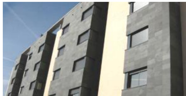
Fig. 7. Facing with facade porcelain stoneware
