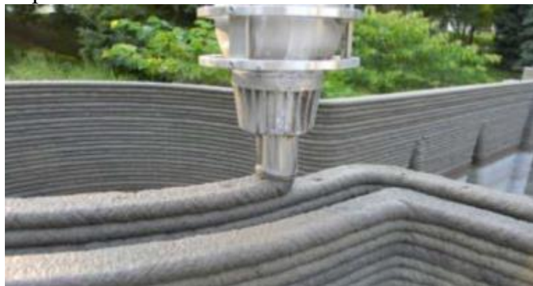
Fig. 3. 3D Construction Process Using the Concrete Printing Technology [1]
