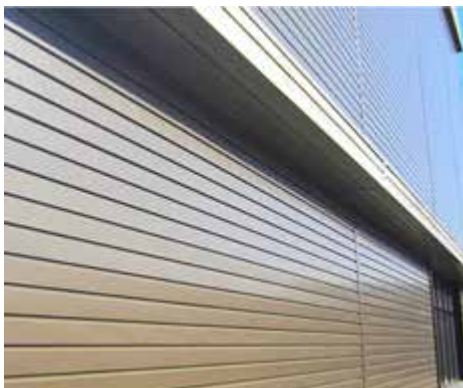
Fig. 4. Facade decoration with siding
