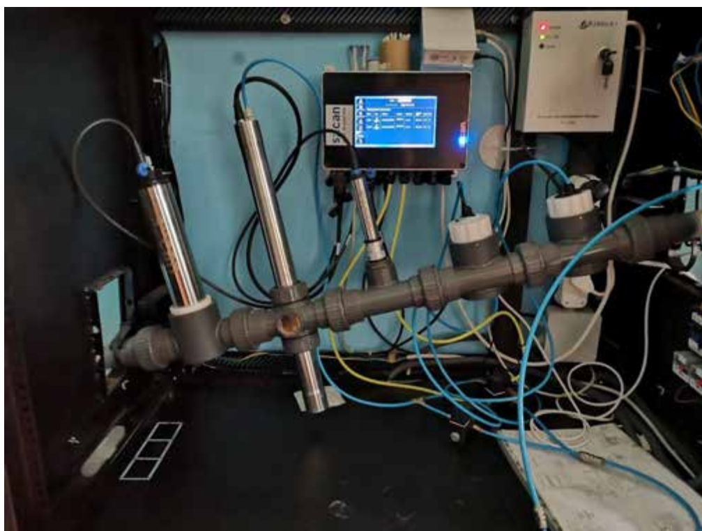
Figure 5.1 Monitoring of water quality through automated environmental monitoring system: APS 9701 - Hydropost 1. Sviatohirsk, February 2020. Source: Communal enterprise of Donetsk oblast council "Environmental Monitoring Centre"
