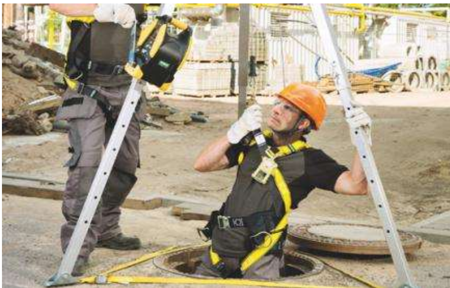
Fig.1. The work in closed containers and spaces
