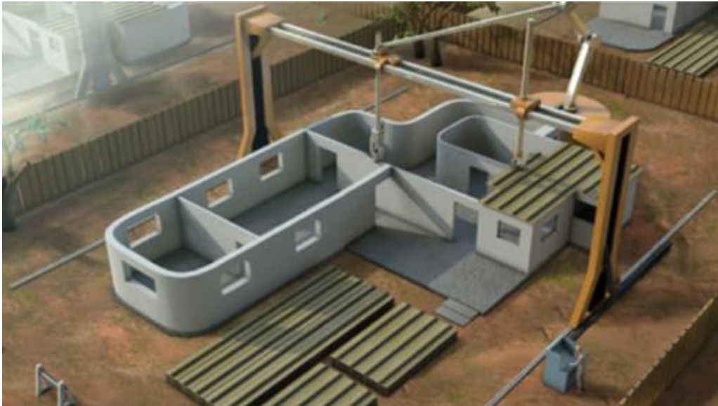
Fig. 2. 3D Printing Setup for Building Construction Using the «Contour Crafting» Technology [1]
