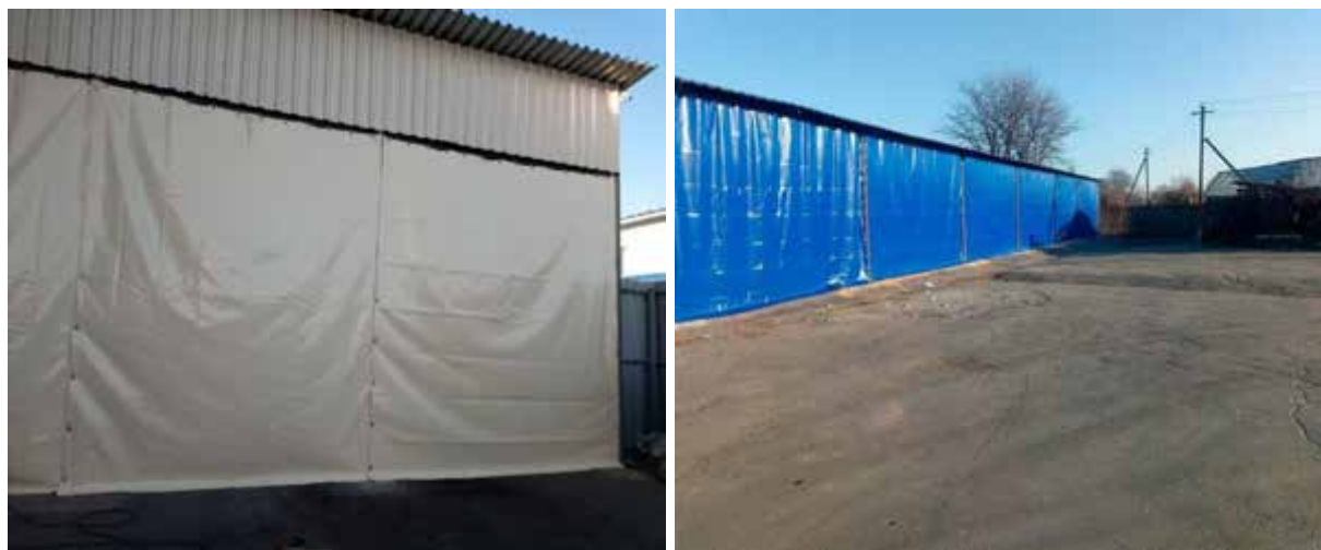
Fig. 1. Equipped storage shed for harvesters.
