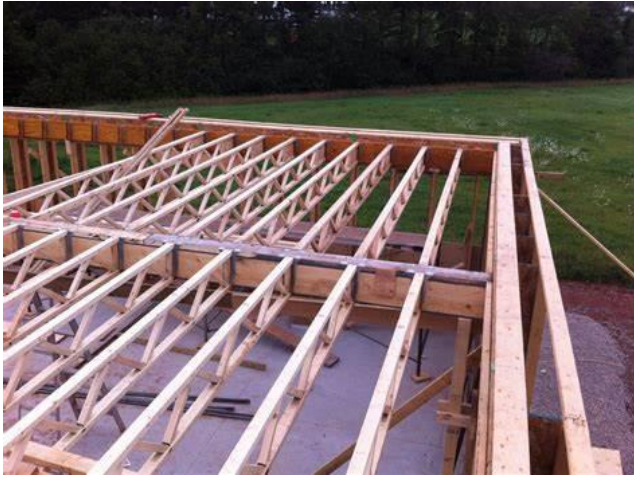
Fig. 2.2. The installation of trusses like as floor constructions.
