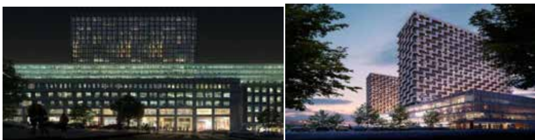
Fig. 4. Renovation project in Kiev
