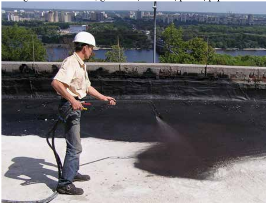
Fig. 2. Mechanical application of bitumen mastic
