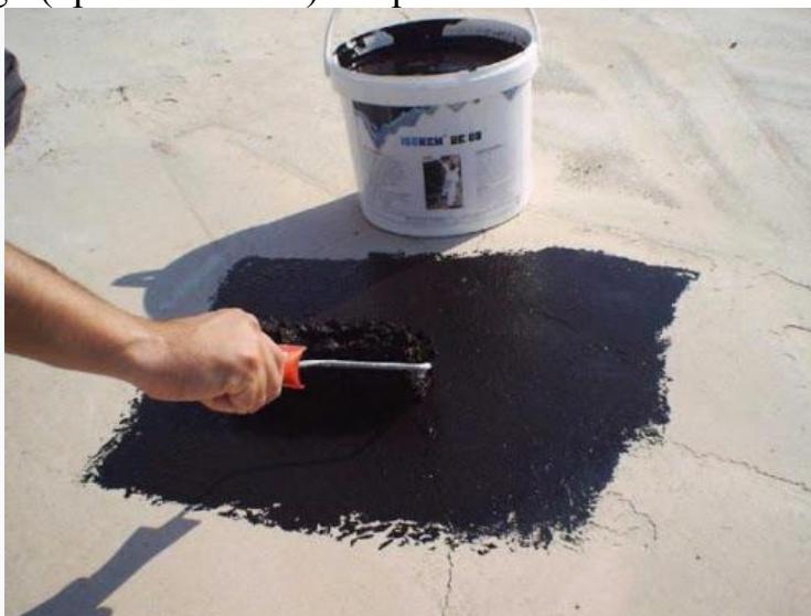
Fig. 1. Manual application of bituminous mastic
